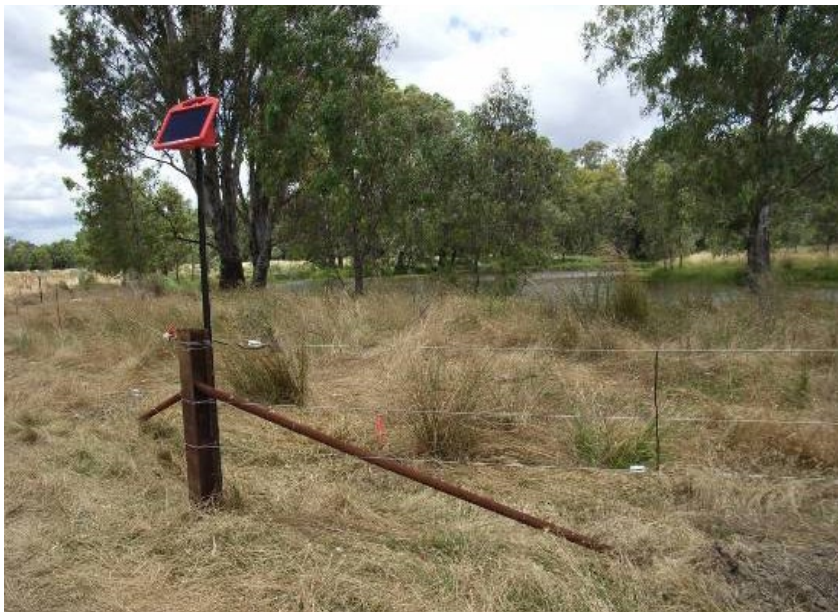
Image 3: Flood fencing installed on a billabong wetland (see map on page 33 for photo location). The design incorporates very strong railway iron end assemblies with a minimal fence panel construction of three electrified plain wires. The widely spaced plain wires are less prone to collecting flood wrack which is the usual cause of fence damage during floods. The use of timber 'droppers' also helps by making the fence panels very flexible (the panel can twist). Each section of fence between the railway iron posts is also wired separately – this ensures that if one section is washed out it doesn't take the rest of the fence with it.
