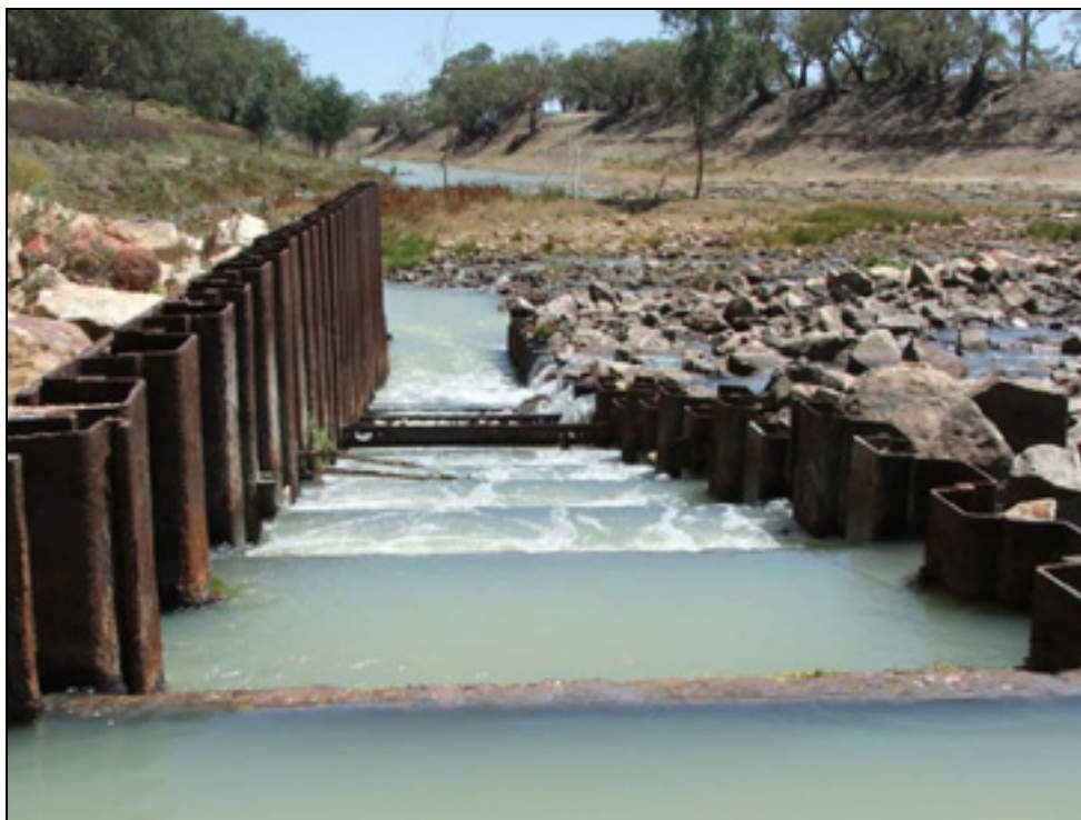
Figure 2. Submerged orifice fishway, Tilpa Weir (No. 24), Darling River (02.12.2004, 144.6ML/day).
