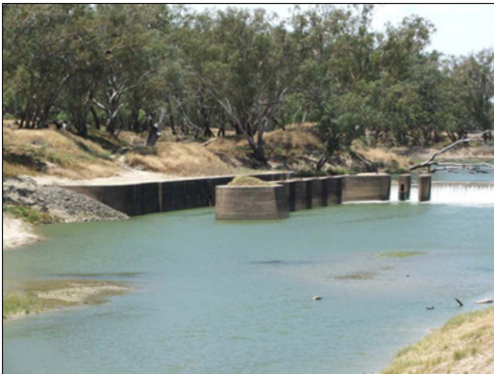
Figure 2. Defunct boat lock, Bourke Weir, Darling River (01.12.2004, 144.6ML/day).
