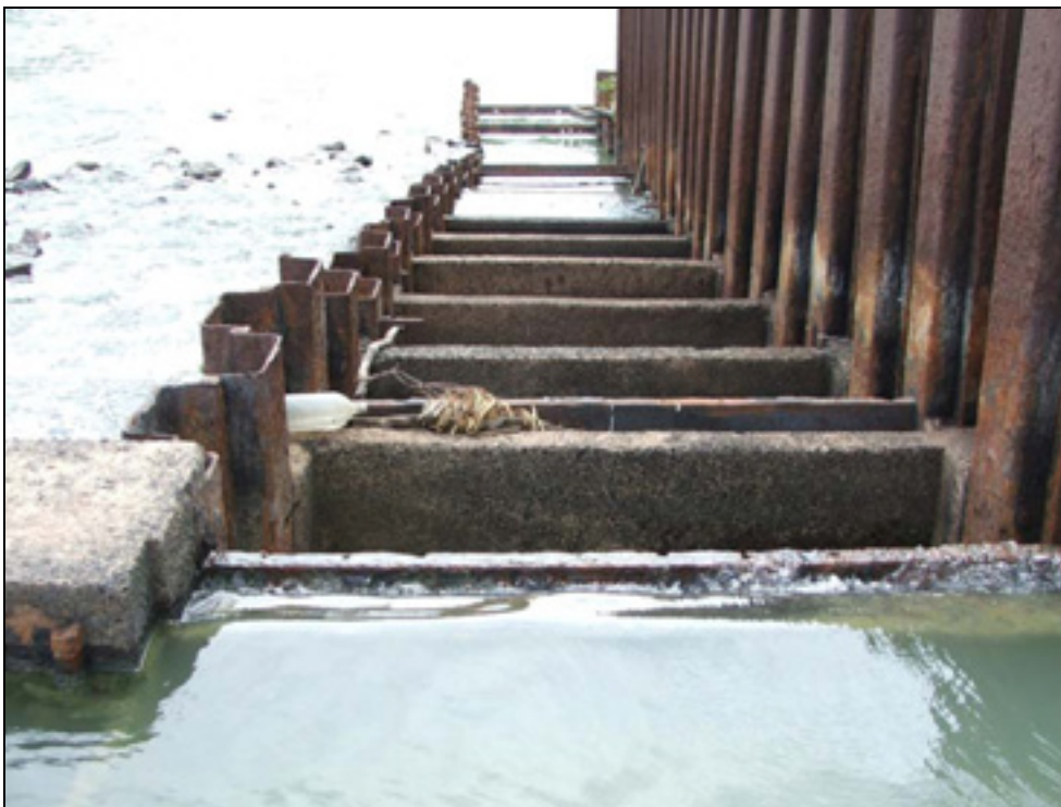
Figure 2. Defunct fishway, Weir 19A, Darling River (01.12.2004, 144.6ML/day).
