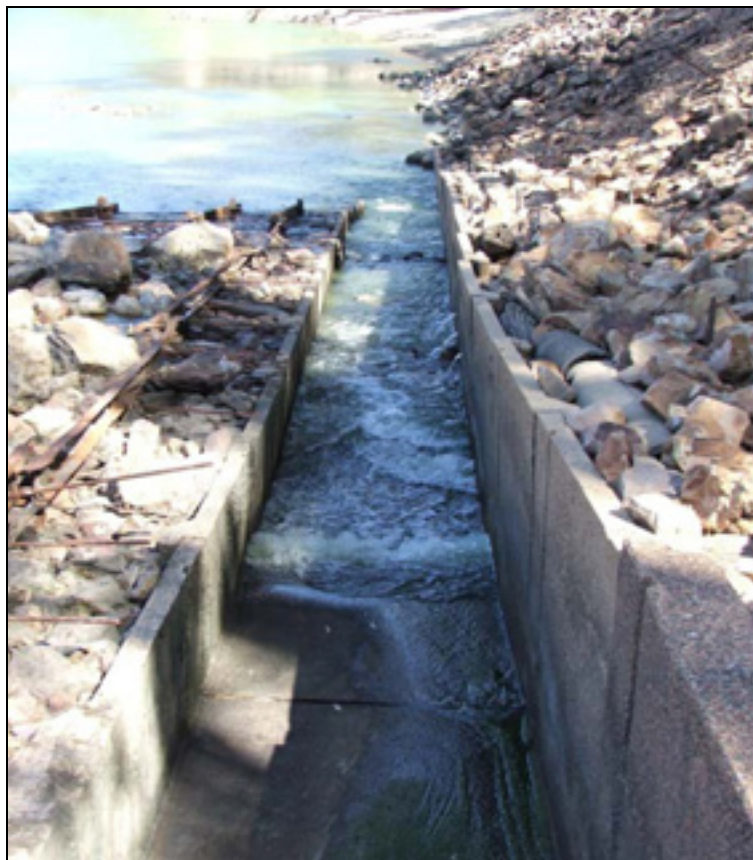
Figure 2. Submerged orifice fishway, Louth Weir 21, Darling River (02.12.2004, 144.6ML/day).
