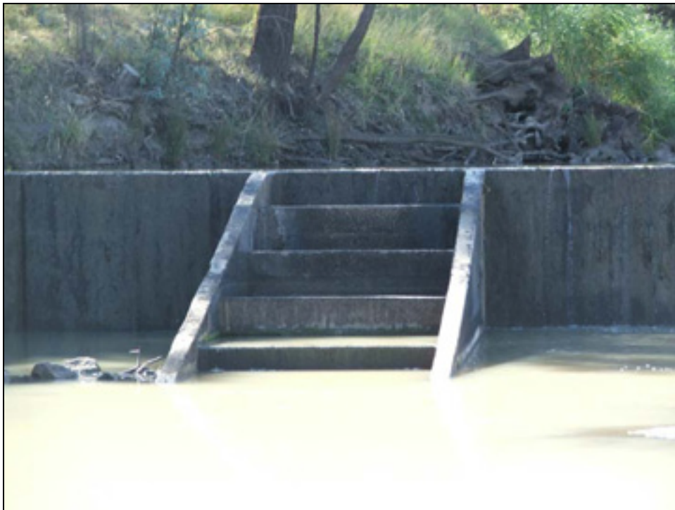
Figure 2. Submerged orifice fishway, Collarenebri Weir (No. 5), Barwon River (16.05.05, 8.7ML/day).
