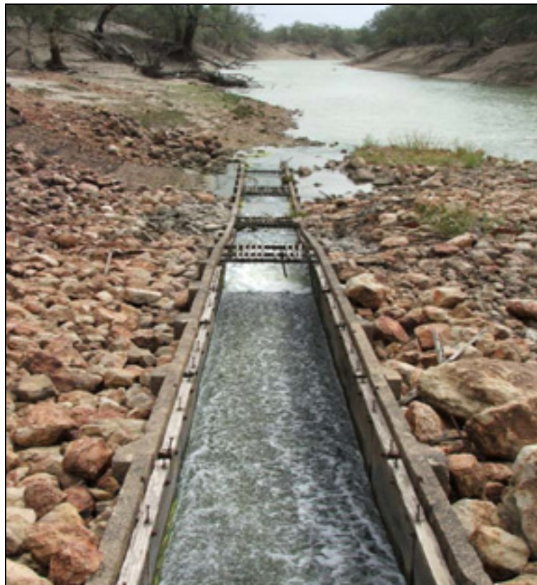
Figure 2. Submerged orifice fishway, Weir 20A, Darling River (02.12.2004, 144.6ML/day).
