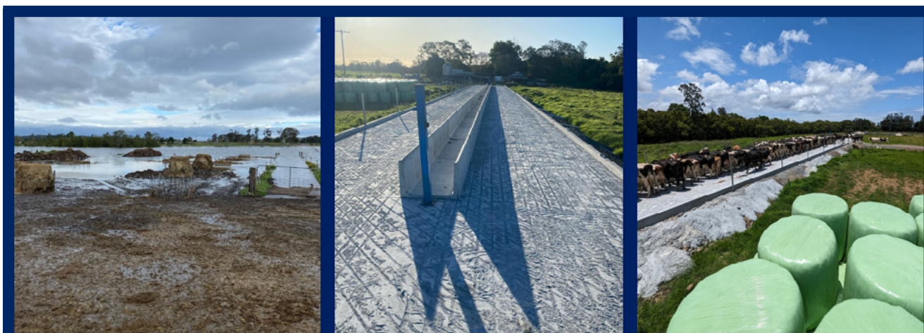
Evolution of a flexible feeding system- from gravel mounds and hay racks to concrete feed pad in 18 months.
