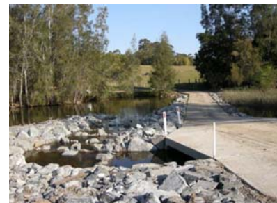
Post works – reinstated fish passage. Photo I&I NSW
