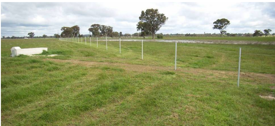
Image 16: Troughs installed and fence under construction, July 2007.
