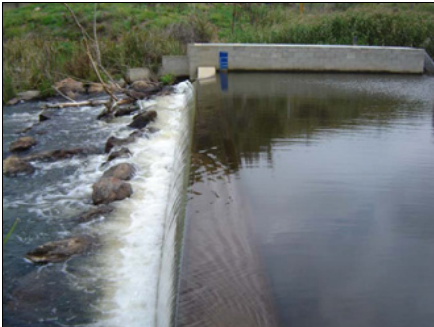
Figure 2. Vertical slot fishway on right abutment of Dalgety Weir. Note wood debris blocking downstream rock ramp fishway approach and vertical slot fishway entrance (3/03/05, 98ML/day).
