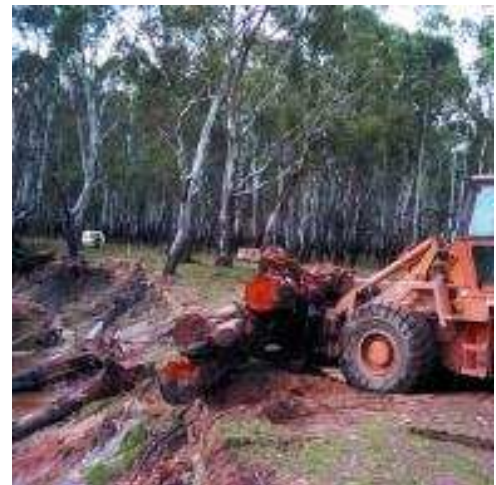
Figure 6: A rubber tyred front end loader is a more sensitive method of putting snags into place on the bank (photo: ARI)
