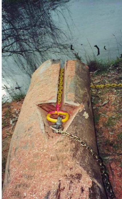
Figure 8: Quick release mechanism - a fast and efficient method of dragging snags into place (photo: ARI).
