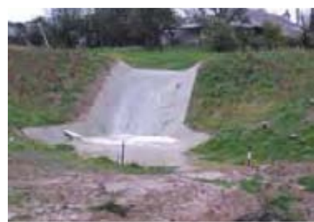
Lining a degraded drainage line with rocks to prevent further erosion (above) A cement flume, preventing erosion associated with dam overflow (below) (Photos courtesy of the Hawkesbury-Nepean Catchment Management Authority)
