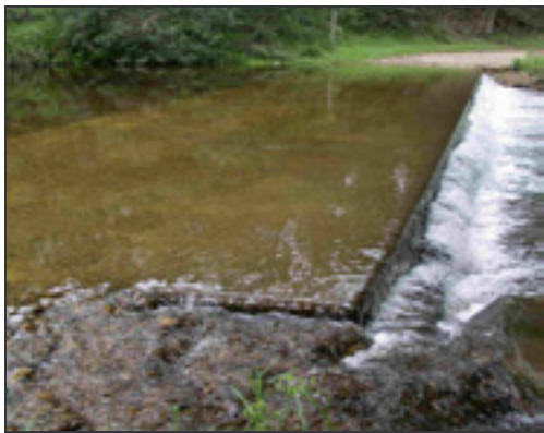
Photo 1. Causeway with high invert (headloss) and shallow water depth (Currowan Ck, Eurobodalla subregion)
