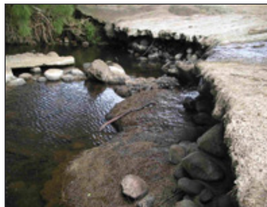
Photo 4. Scoured causeway creating a large headloss (Sawyers Ck, Shoalhaven/Wollongong subregion)
