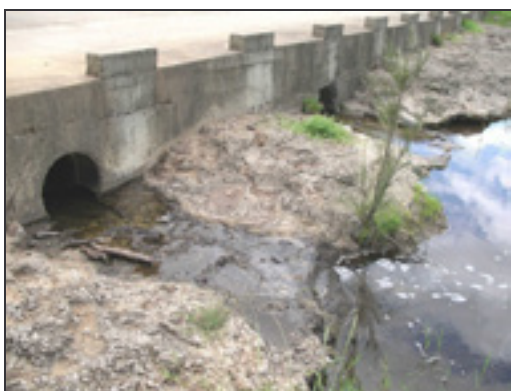
Photo 3. Piped causeway with inadequate sized pipes, high invert (headloss) and shallow water depth (Bettowrynd Ck, Eurobodalla subregion)
