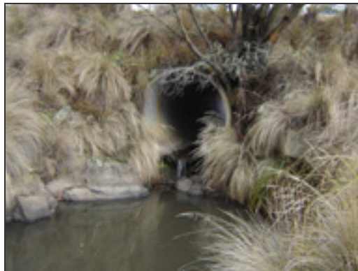
Photo 2. Pipe culvert with high invert (headloss) (Black Swamp Ck, Snowy subregion)
