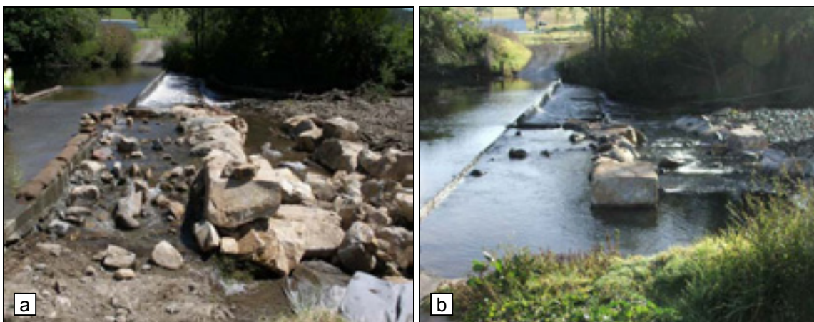
Figure 5. Faulkland Road Crossing modified partial width rock ramp fishway (a) during construction, (b) completed work.
