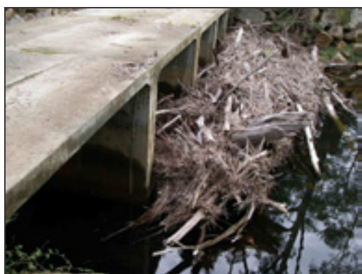
Photo 11. Box culvert with woody debris (Stony Ck, Eurobodalla subregion)
