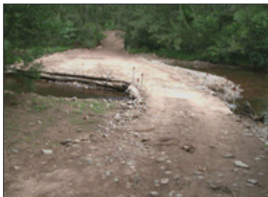
Photo 6. Earth levee with inadequate sized pipes creating velocity barrier (Deua R, Eurobodalla subregion)
