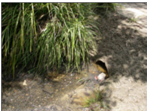
Photo 9. Pipe culvert of inadequate size and large sediment inputs (Duck Ck, Eurobodalla subregion)
