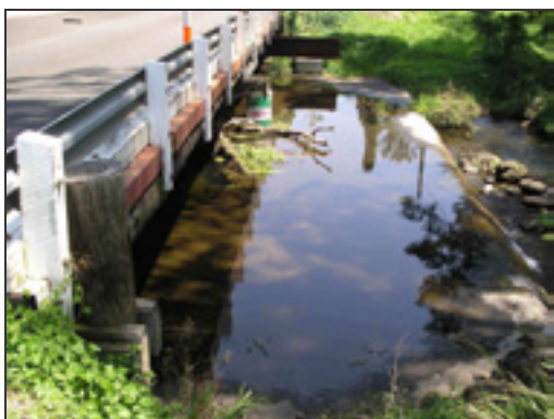
Photo 7. Redundant causeway used as bridge base, high invert (headloss) and shallow water depth (Frys Ck, Shoalhaven/Wollongong subregion)
