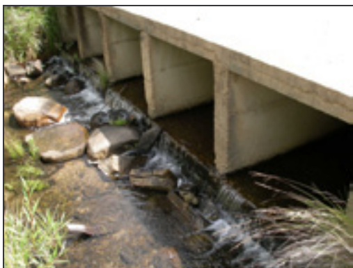
Photo 5. Box culvert with high invert (headloss) and shallow water depth (Jinden Ck, Shoalhaven/Wollongong subregion)
