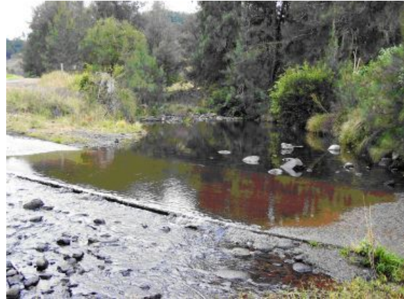
Road crossing restricting fish passage
