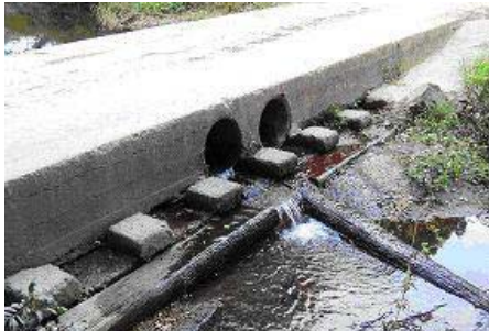
Before & after photos of the same road crossing rehabilitated to allow safe fish passage
