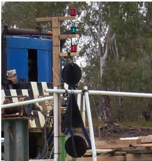
Figure 7 (left): Floating Barge with Channel Blocked day shapes and night-lights.
