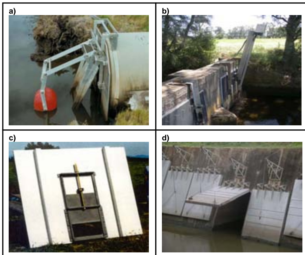
Plate 1: Examples of floodgate modification designs including a) tidal floodgate, b) 'Smart Gate', c) sluice gates, and d) winch gates.
