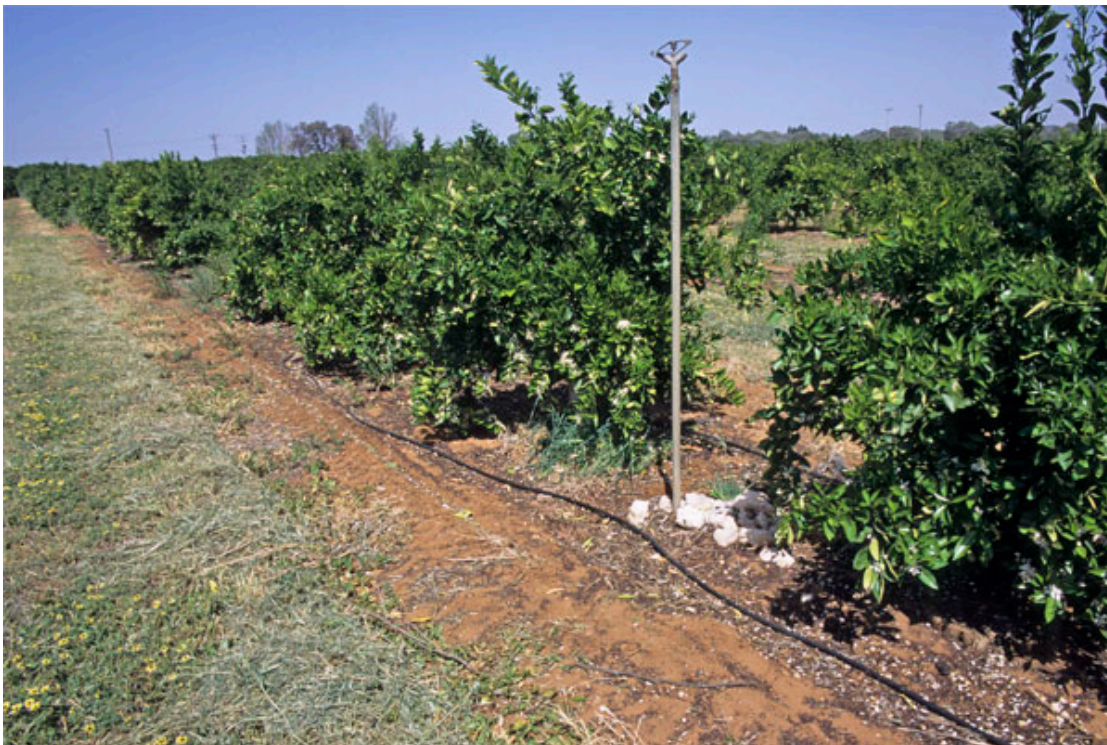
Figure 1. Overhead sprinklers are retained in a recently installed drip orchard.
