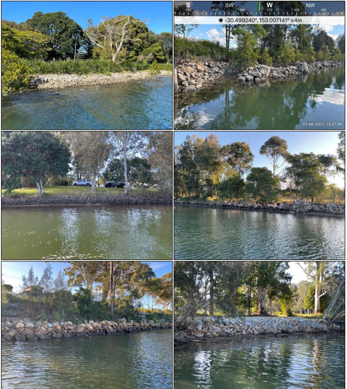
Plate 14 Examples of effective bank protection works in the study area, clockwise from top left: Cobble beaching in lower Kalang River Reach 268; Rock fillets at Newry Island, Kalang River Reach 662; Large woody debris/rootballs in the lower Kalang Reach 739; Rock armouring adjacent to Yellow Rock Road on Back Creek Reach 353; Rock armouring and logs at Mylestom on Bellinger River Reach 355; Gabion wall at Mylestom on the Bellinger River Reach 29.
