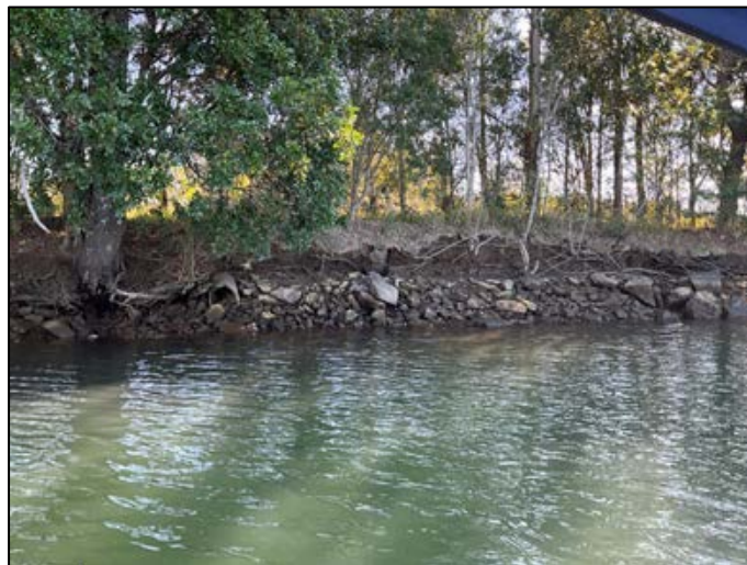
Plate 16 Examples of partially effective bank protection works (condition) in the study area, from left to right: erosion of the mid bank above slumped rock armouring in the lower Bellinger River Reach 57; subsiding rock works on Back Creek exposing upper bank to erosion, Reach 723.
