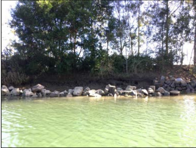
Plate 15 Examples of partially effective bank protection (design) in the study area, from left to right: insufficient rock fillet height and subsequent erosion of the mid bank on the Kalang River Reach 654; failure of the bank toe and subsequent subsidence of rock armouring on the Kalang River Reach 660.
