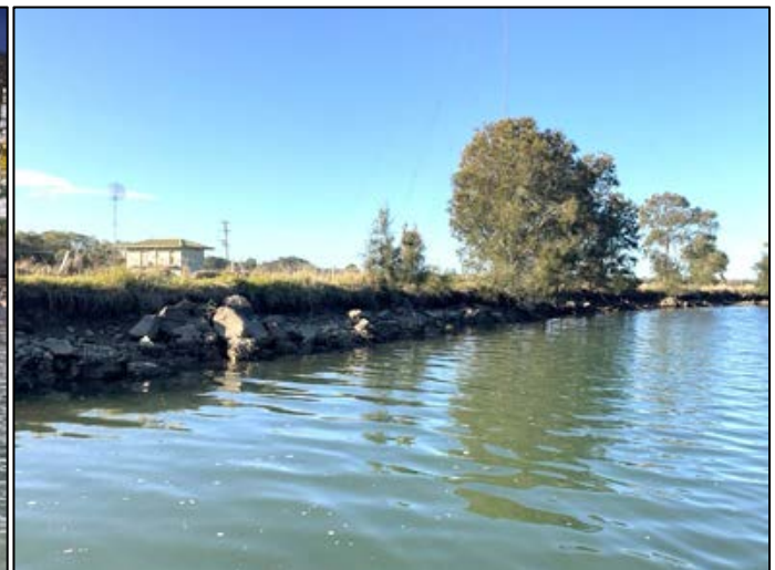
Plate 16 Examples of partially effective bank protection works (condition) in the study area, from left to right: erosion of the mid bank above slumped rock armouring in the lower Bellinger River Reach 57; subsiding rock works on Back Creek exposing upper bank to erosion, Reach 723.
