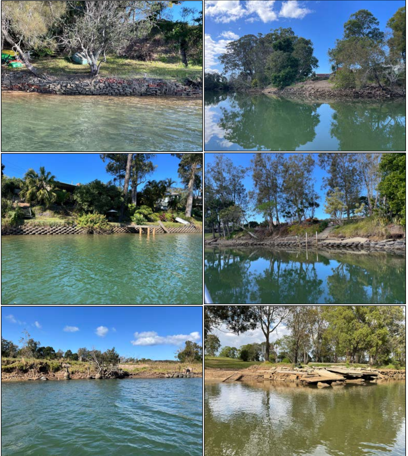
Plate 17 Examples of inappropriate bank protection works in the study area, clockwise from top left: building rubble dumped over the bank at Reach 261 Kalang River; building rubble pushed over the bank on the Council reserve at Reach 333 Kalang River; tyre wall in the Council reserve area behind Burrawong Pde Kalang River; Concrete debris and building waste on the Kalang River; deteriorating tyre wall Kalang River Reach 425; tyre wall on the Bellinger River at Raleigh Reach 77.
