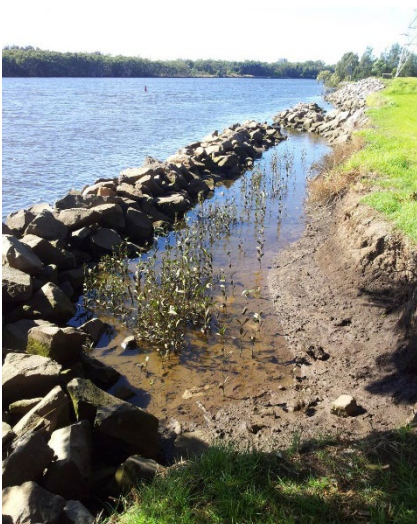
Figure 8 Mangrove seedlings establishing on an eroding bank when protected by rock fillets (Photo: Kylie Russell).
