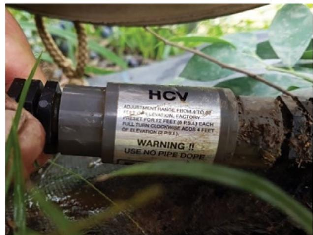
Figure 1. Check valves can reduce the drainage from mains to the lowest dripper. Photo: Robert Hoogers.
