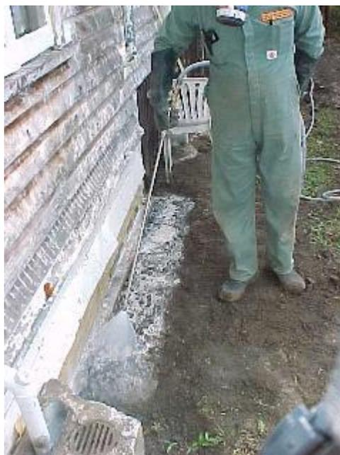
**Figure 5. Termiticide application to a building perimeter by trenching and treating the backfill.**
