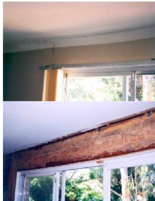
*Figure 3.* Sagging cornices and warping plasterboard (top) can be indicative of termite activity underneath (bottom).
