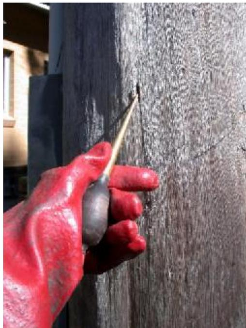
*Figure 4. Termite dusting an infested power pole.*
