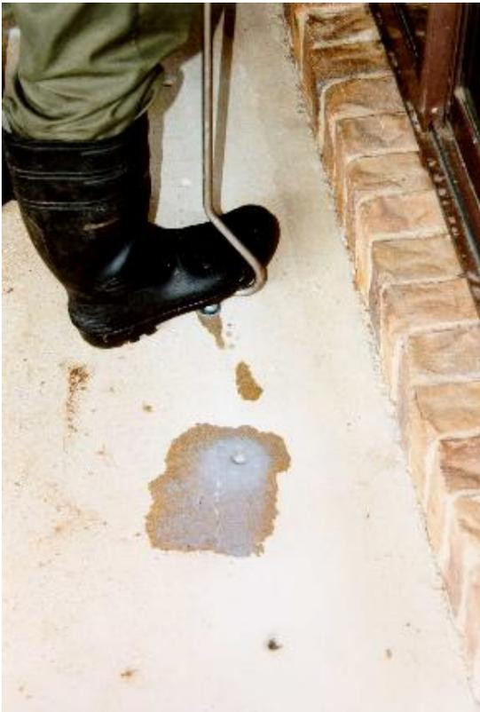
Figure 6. Injecting termiticide through holes drilled in a slab. Holes are sealed after treatment.
