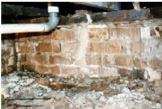
**Figure 2.** Main gallery by which termites enter a building. A nearby leaking water pipe probably encouraged termites into this part of the building.
