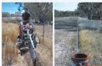
Riparian fencing and laying pipe for watering troughs (2006).
