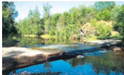
Quart Pot Crossing before fish passage works (2005).
