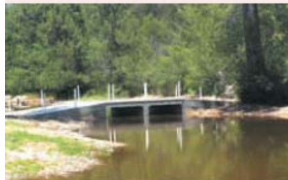
Quart Pot Crossing after fish passage works (2006).
