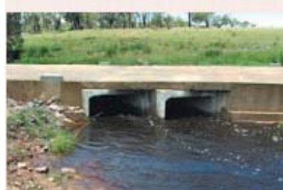
Crossing after the installation of fish friendly box culverts (2006).
