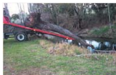
Snag being placed at Molong Creek site.
