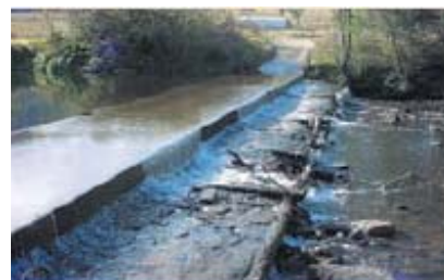
Barrier to fish passage on the Gloucester River prior to fish passage works taking place (2004).
