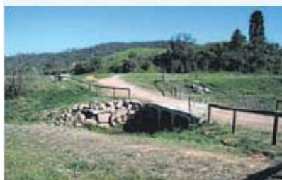
Crossing, fencing and erosion protection works completed November (2006).
