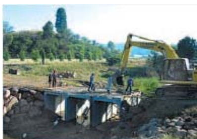
Construction of fish friendly crossing, March (2006).
