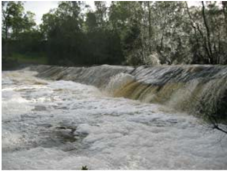
The Branch River Crossing during flood - note height of the structure. Photo: C. Thrupp.
