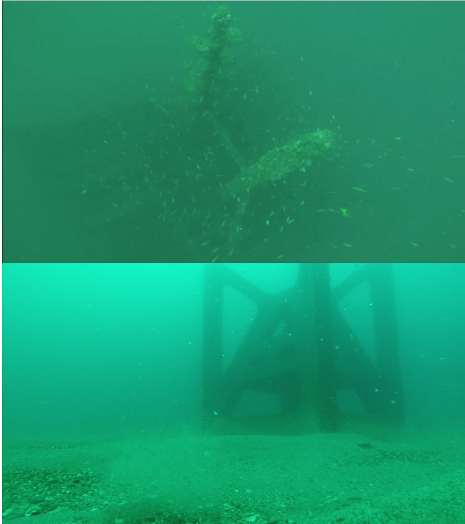
Figure 21 Inspections of the Sydney (upper image - 7 May 2015) and Shoalhaven (lower image - 18 May 2015) OARs following an intense east coast low that produced waves up to 15 m (Hmax)
