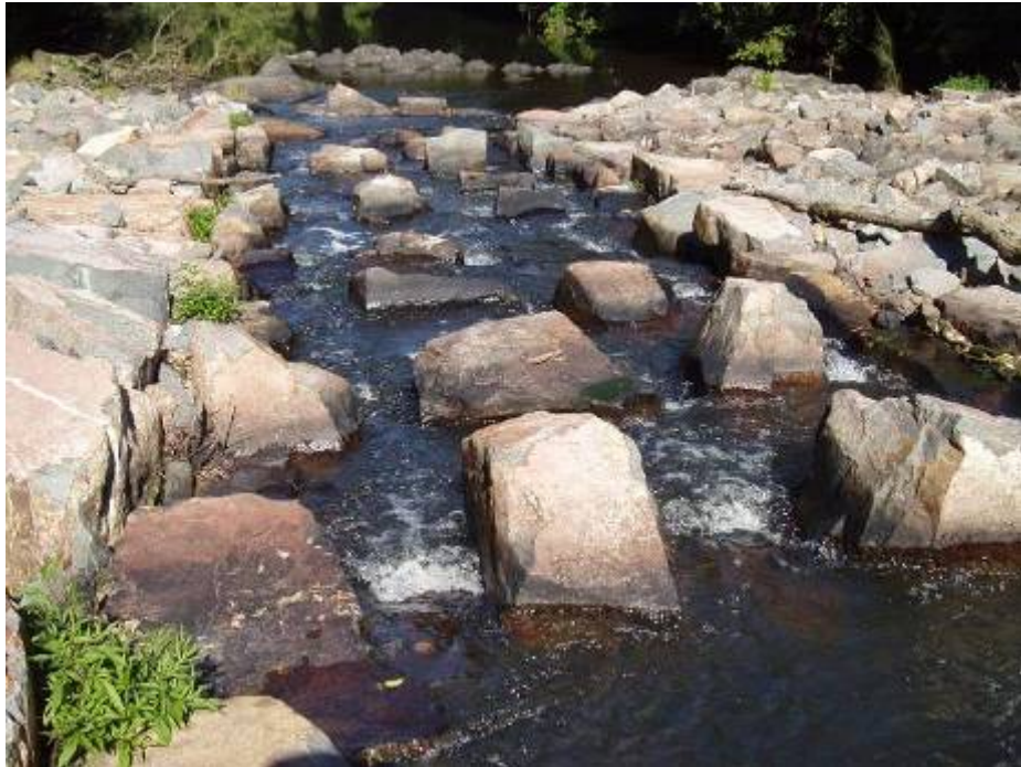
Figure 17. Low-flow fishway located within the full width rock ramp showing flows characteristic of those sampled during this study.
