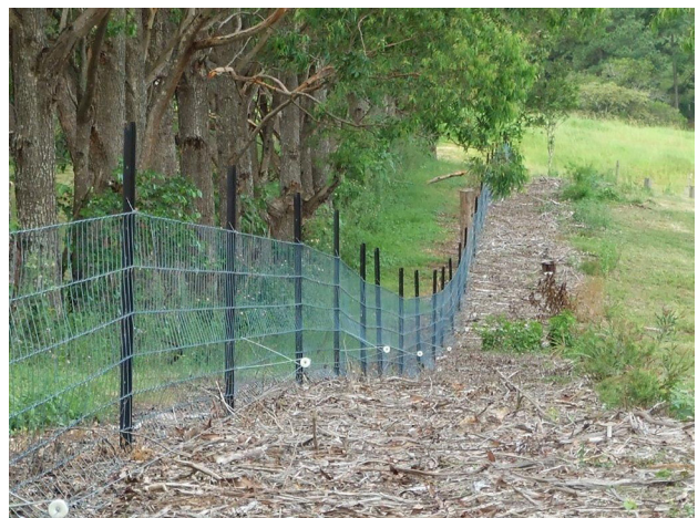
Figure 5. An effective pig exclusion fence.
