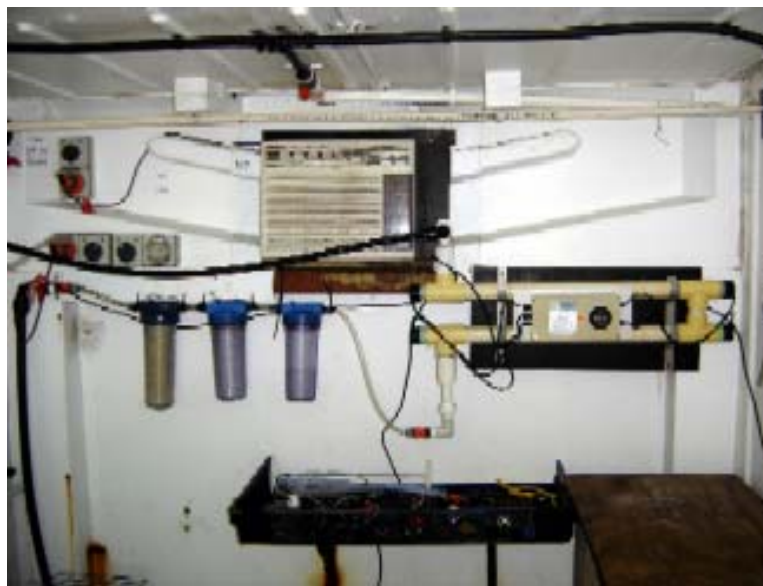
Fig 8. Three cartridge filters and the UV sterilisation unit in line with the seawater supply hose.
