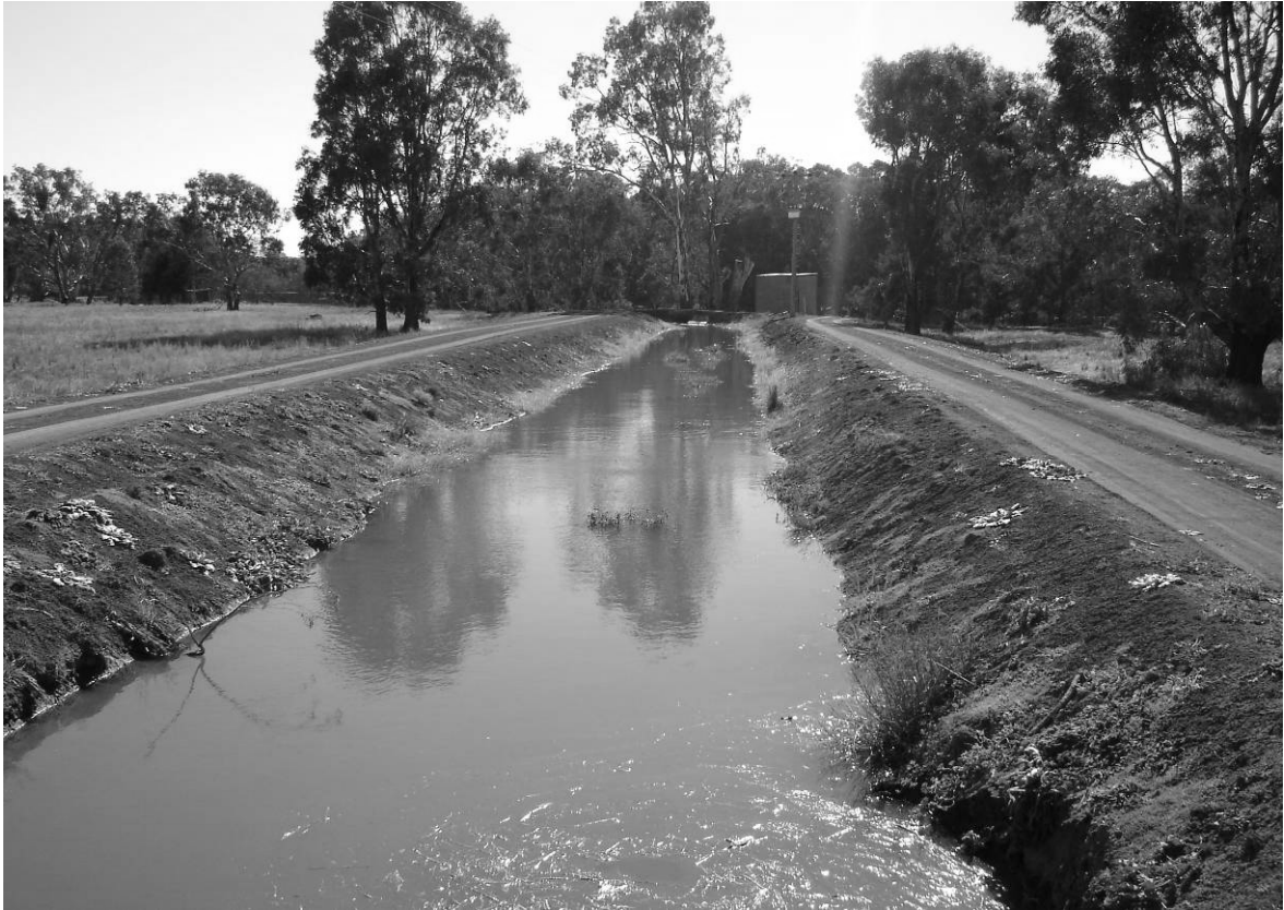
Figure 1.1. A gravity-fed irrigation channel typical of those constructed in the Southern reaches of the Murray-Darling Basin.
