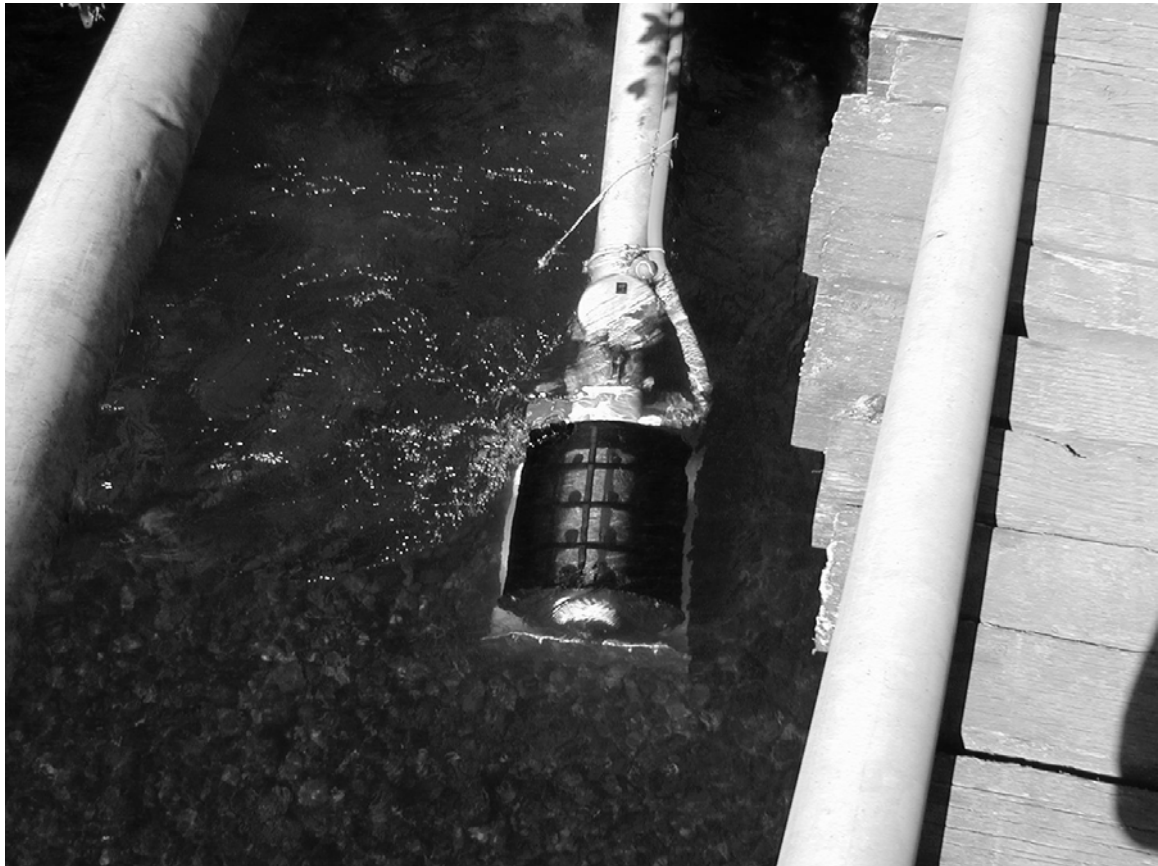
Figure 6.5. An example of a cylindrical cone screen adapted to fit over the intake of a pump system on Mill Creek, Oregon (USA). ( Photo courtesy of Oregon Department of Fish and Wildlife ).
