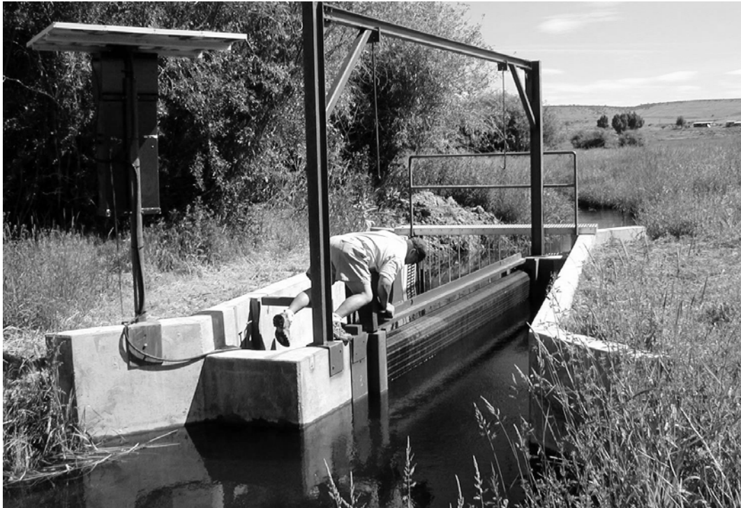
Figure 6.1. A vertical travelling screen commonly used in the USA to prevent fish entrainment into irrigation canal systems. (Photo Courtesy of Oregon Department of Fish and Wildlife).
