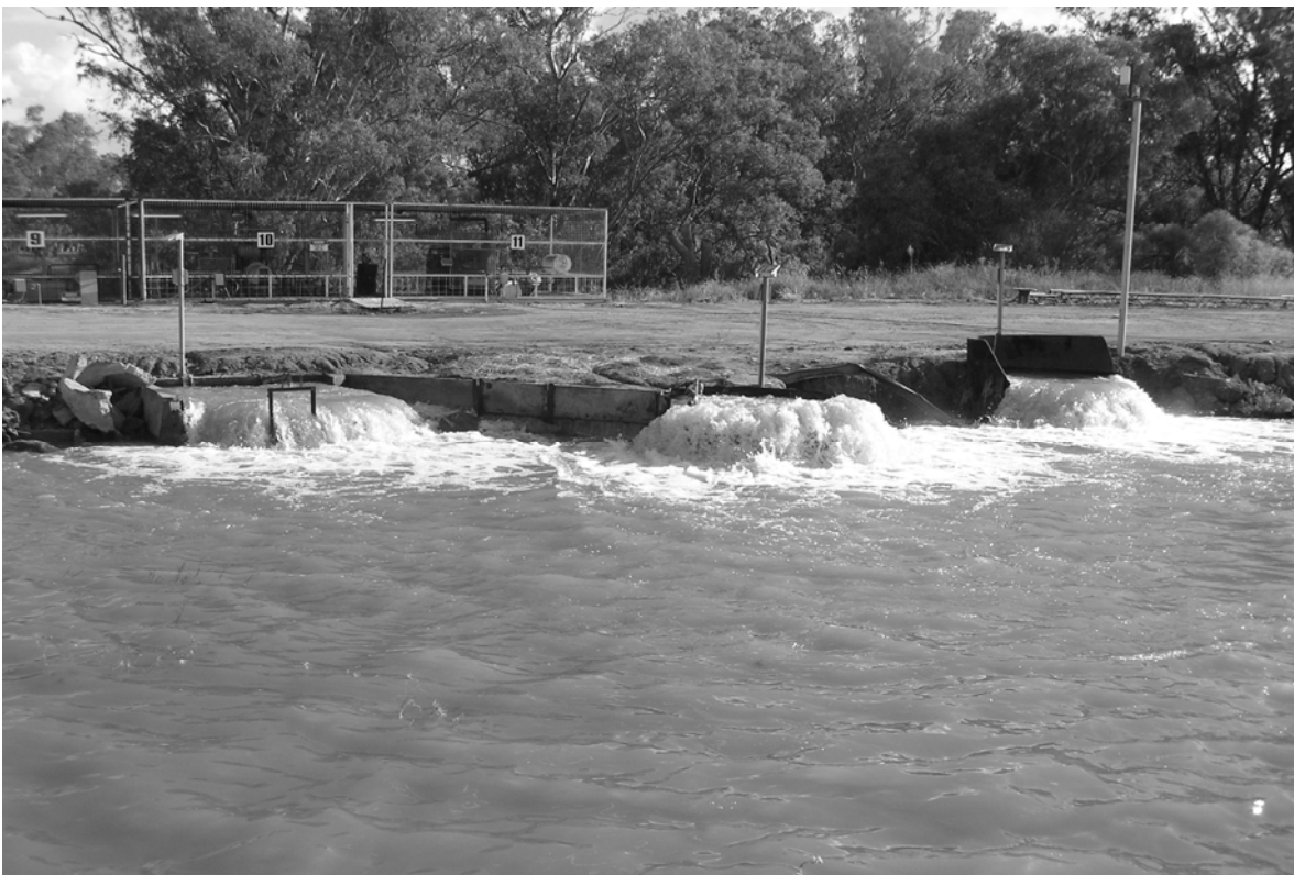
Figure 1.2. An indication of extraction rates from a direct pumping system typical of those constructed in the Northern reaches of the Murray-Darling Basin.
