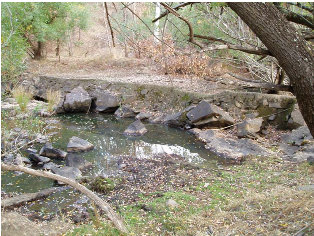
Figure 9. An artificial barrier on Coppabella Creek (-35.79412S 147.69676E) which is believed to exclude redfin perch from 73 km of habitat occupied by southern pygmy perch.
