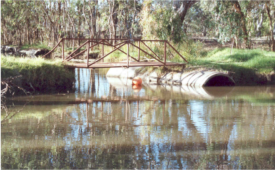
Trapping Site 3. The trap at this site was set and lifted from the bridge; no wings were attached.
