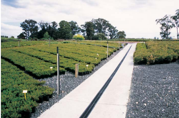
Figure 13. a well-sealed catchment will minimise turbid water
