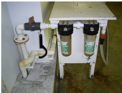
Algae bag and tank filtration through two 1-micron cartridge filters
