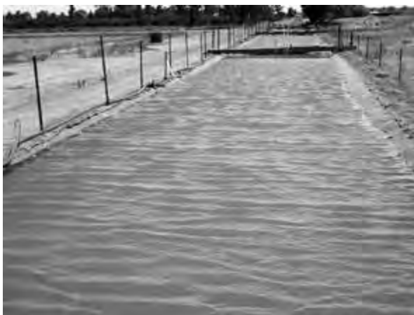
Figure 2. Field setup of lined storages on a commercial irrigation channel.
