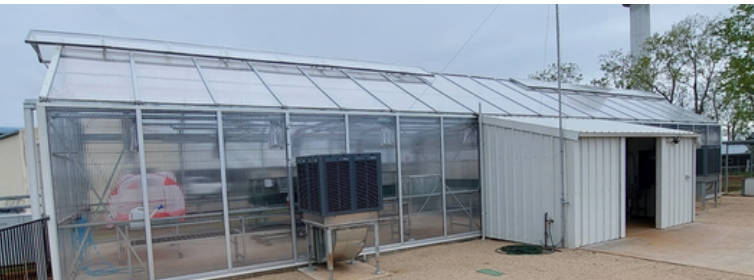
Figure 1: The new fully climate-controlled glasshouse. There are two rooms, with each having independent lighting, roof shutters, internal retractable shade cloth, humidity control, heating, and air-conditioning with both local and remote-control capacity (photo credit Nathan Pugh).
