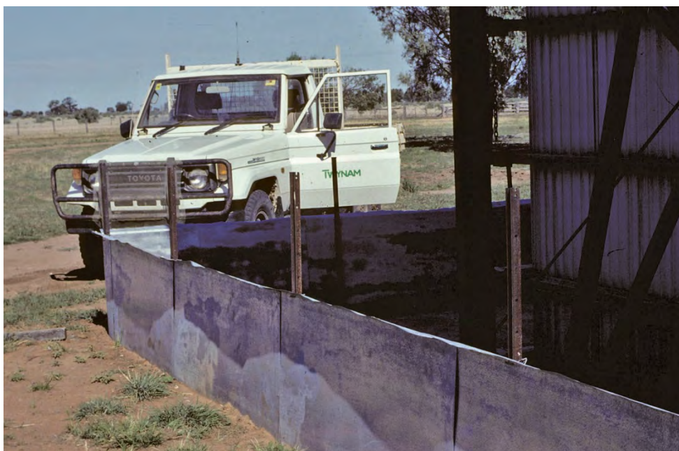
Figure 42. Shed with galvanised barrier (Photo David Croft).
