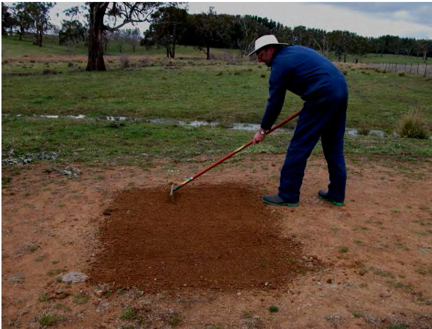
Figure 67: Constructing a sand pad.
