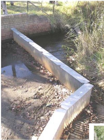
Photo 4: Online GPT, Badoberong Creek, Lower Georges River subcatchment.
