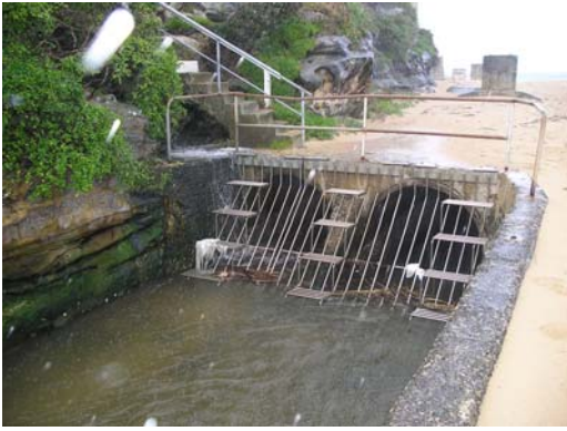
Photo 9: Manly Lagoon outlet structure and online GPT, Northern Beaches subcatchment.
