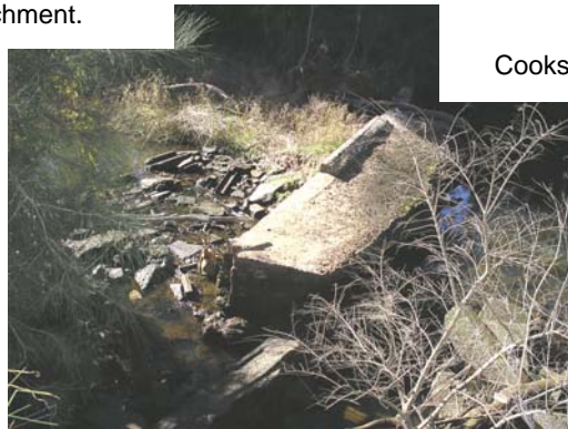
Photo 14: Breached Weir, Cabramatta Creek, Lower Georges subcatchment.
