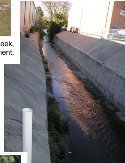
Photo 5: Concrete Channel, Sheas Canal, Cooks River / North Botany subcatchment.
