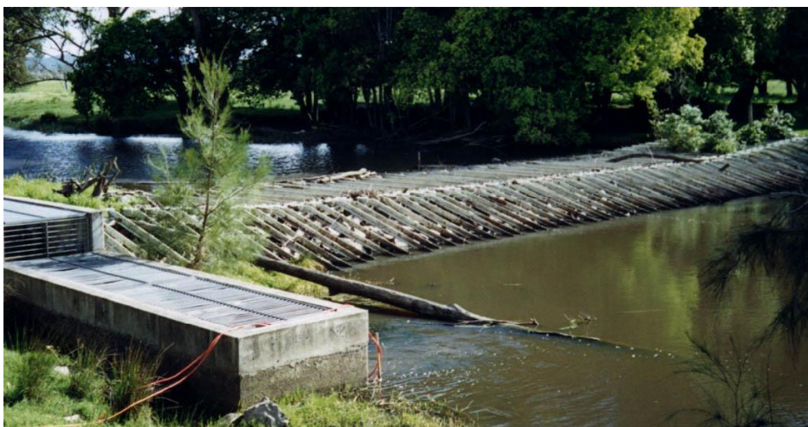
Figure 16. The vertical-slot fishway on the Buladelah Weir. The attracting flow is aligned 90° to the weir face but is approximately 4m downstream. During periods of low flow, the fishway entrance provides the greatest attracting flow although some flow does pass directly through the weir.
