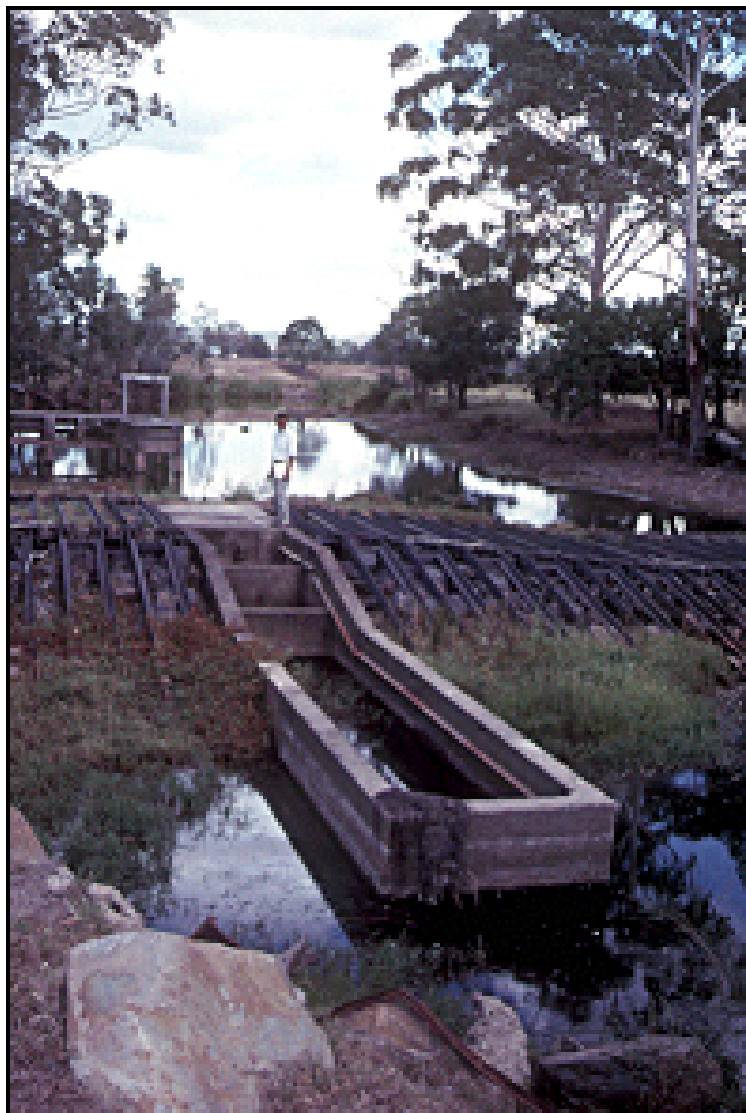
Figure 4. The original (1964) Buladelah fishway. This photo was taken under low flow conditions with the cover grids removed.
