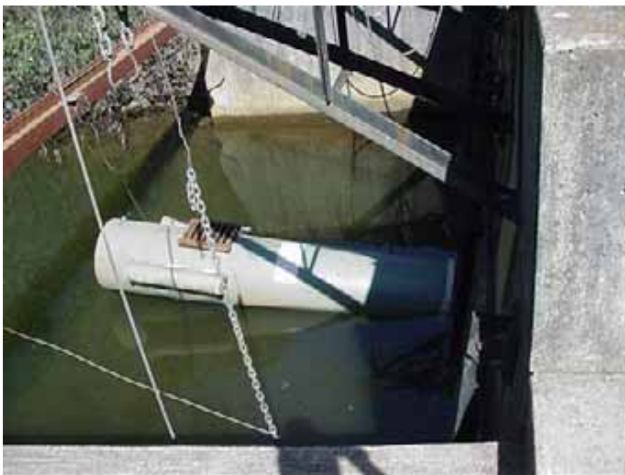
Figure A5.2. Tide-actuated floodgate manufactured by Australian Aqua Services, shown here installed at Oceana Tea Tree.
