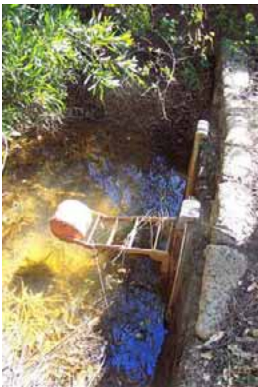
Figure A5.3. Tide-actuated floodgate at Rossglen Drain.
