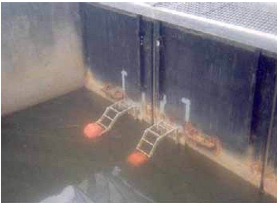
Figure A5.4. Tide-actuated floodgates at Kentwell Farm.
