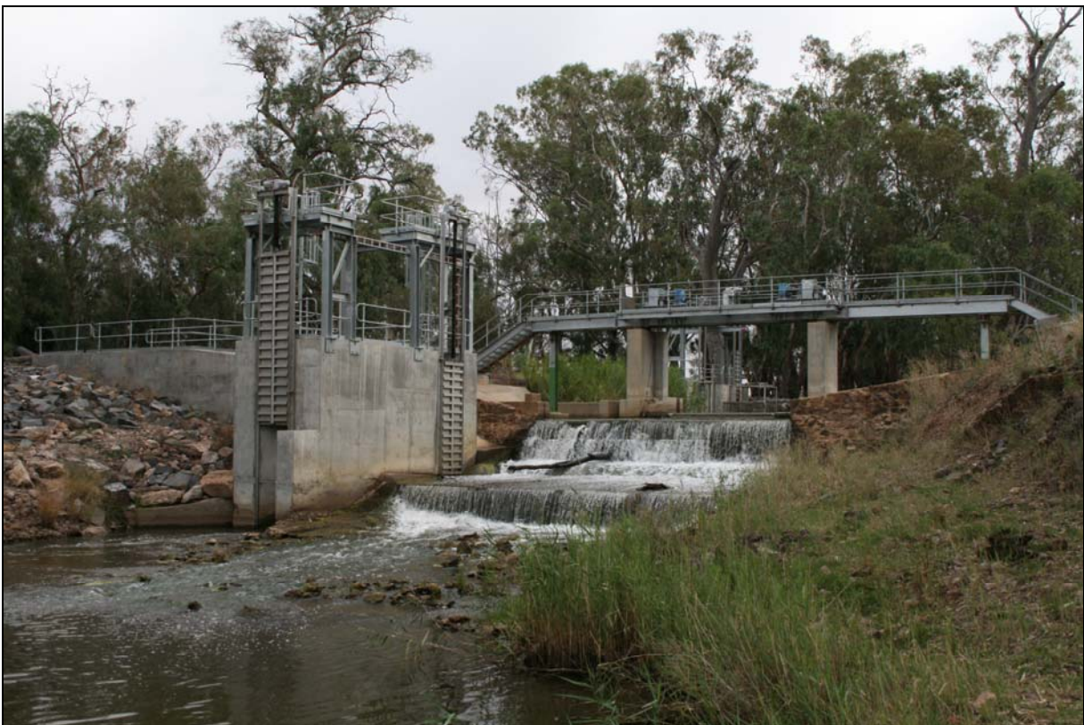
Figure 4.3. The Island Creek Weir and Fishway entrance.
