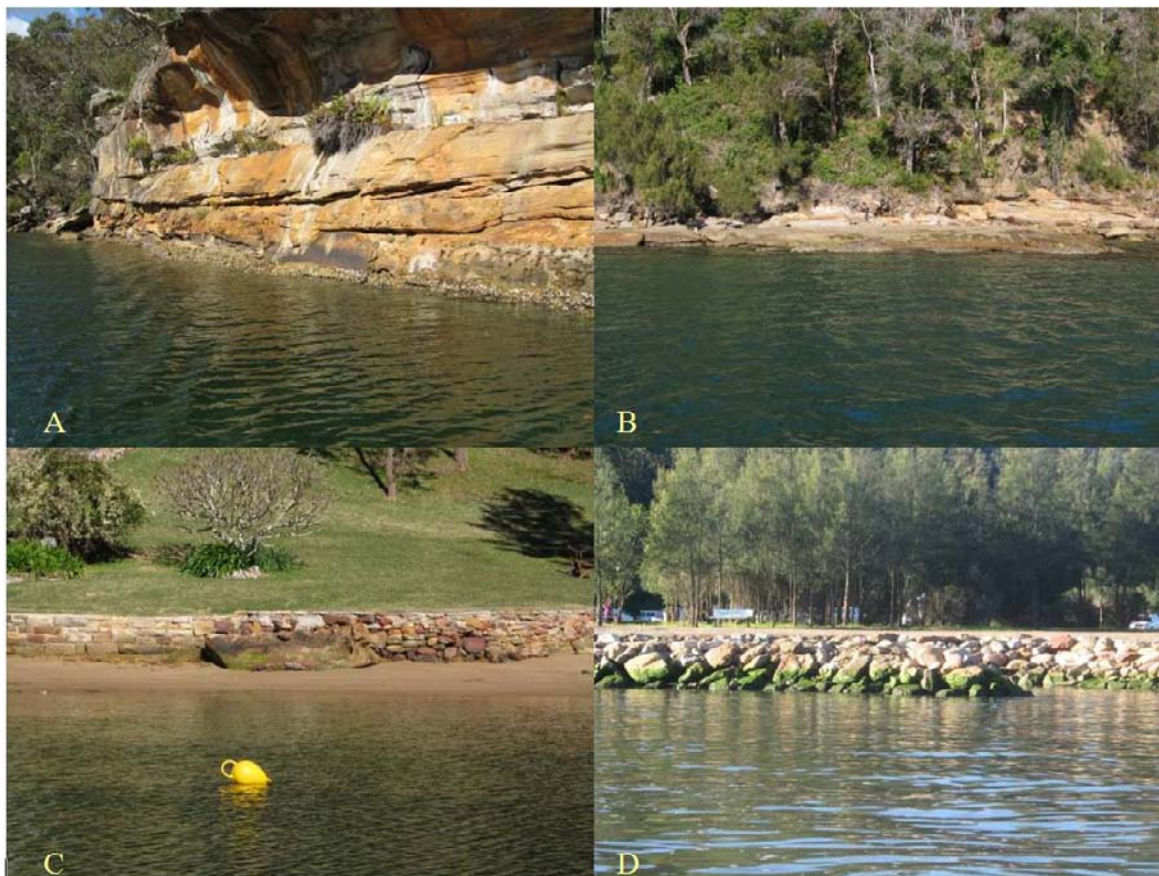
Figure A.4. Examples of hard surface foreshore habitat in the Lower Hawkesbury Estuary. Natural vertical rock platform (A), natural horizontal rock platform (B), artificial rock walls (C&D).
