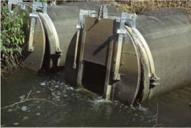
Figure 1: Aluminium sluice gate and floodgate Dungarubba Creek
