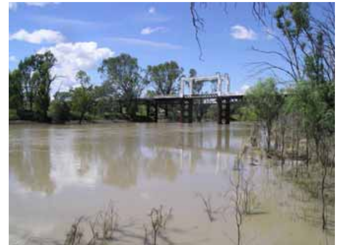
2010 flood levels at the Bourke Bridge. Photo: Scott Nichols.
