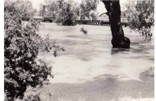
1974 flood levels at the Bourke Bridge. Photo source: Bourke Public Library.
