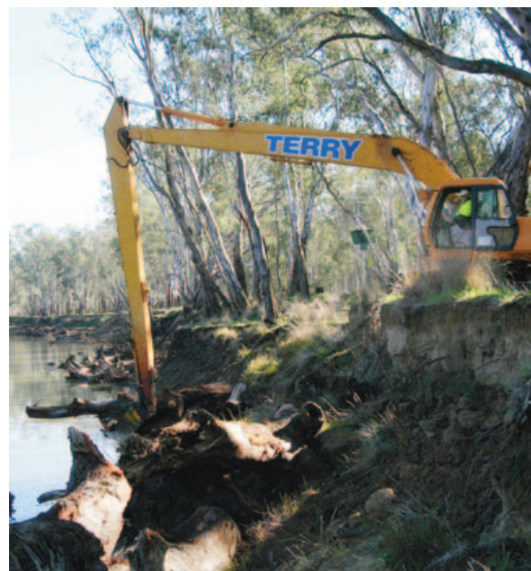
FIGURE 10.3: Snag timber from the Hume Highway Duplication project was placed in the Murray River and now provides habitat for threatened native fish species such as Murray Cod ( Maccullochella peelii peelii ) and Trout Cod ( Maccullochella macquariensis ) (Photo: J Fredrickson, DPI).
