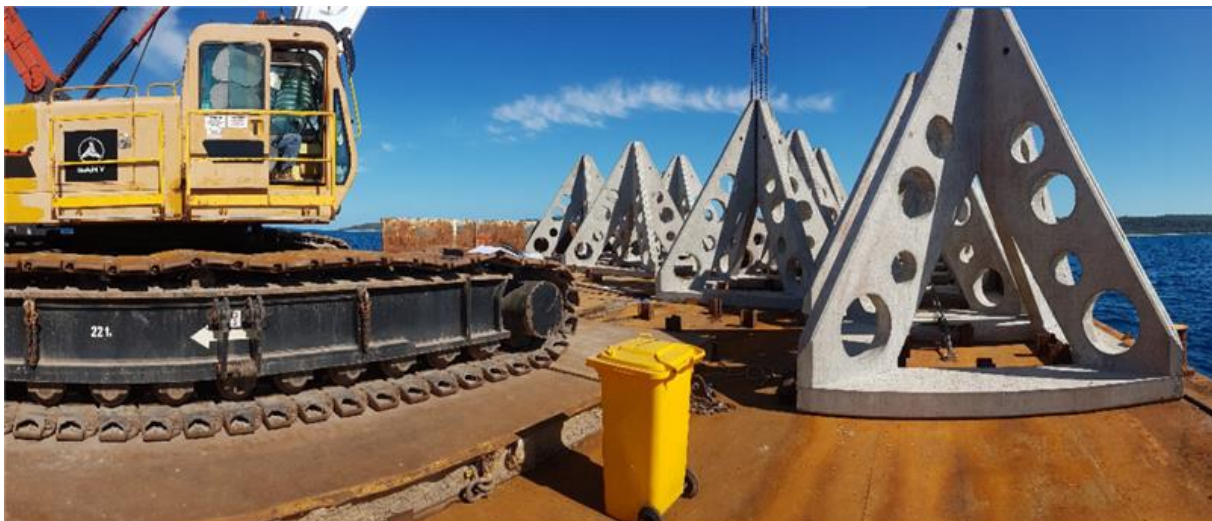
Figure 13 Arrowhead modules used for Stradbroke Island project
