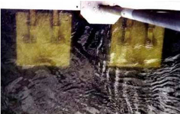
Image 69: open fish flaps attached to penstocks in Swan Creek (Clarence Valley Council)
