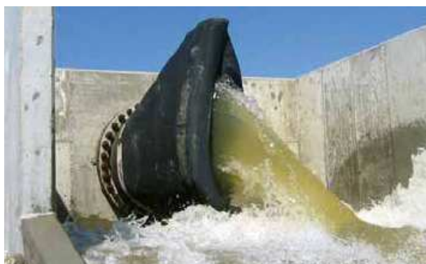
Image 16: elastomer check valves (Fuller Valve)
