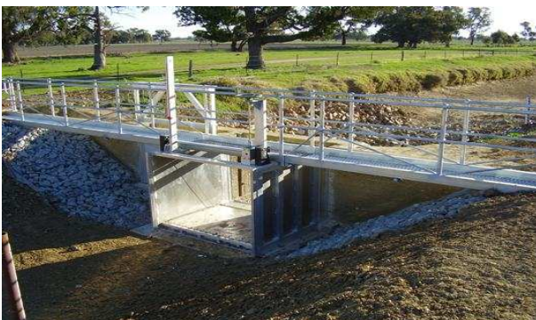
Image 54: single celled lay-flat gate (AWMA)
