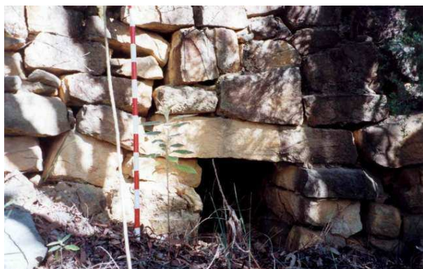
Image 5: sandstone box culvert (NSW RTA)
