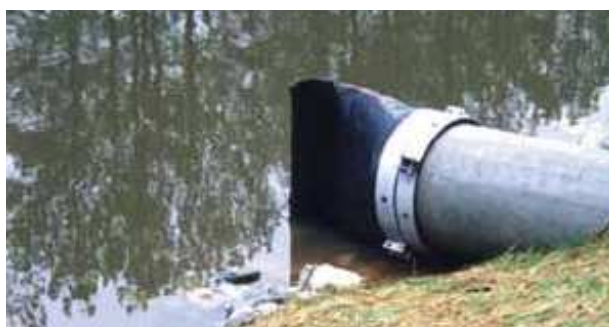
Image 15: elastomer check valves (Tideflex Technologies)
