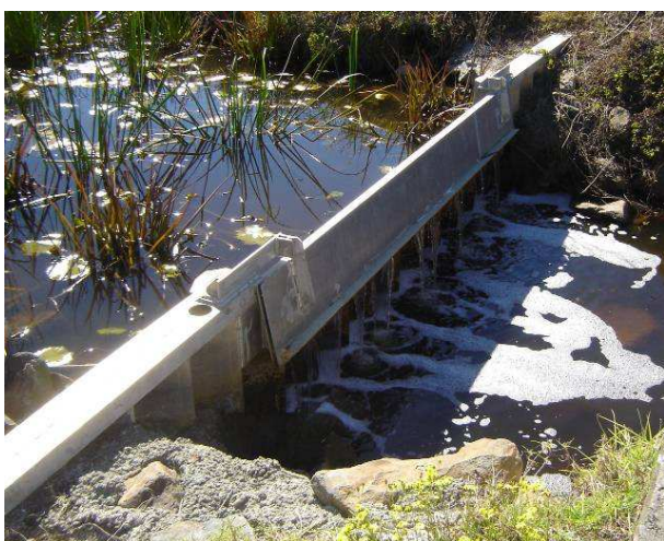
Image 47: pre-fabricated stainless weir with tidal exclusion gate in Port Macquarie
