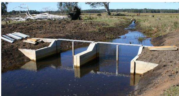
Image 57: installation of precast drop-board weir (S Walsh)
