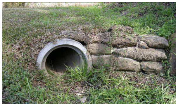
Image 1: single pipe culvert
