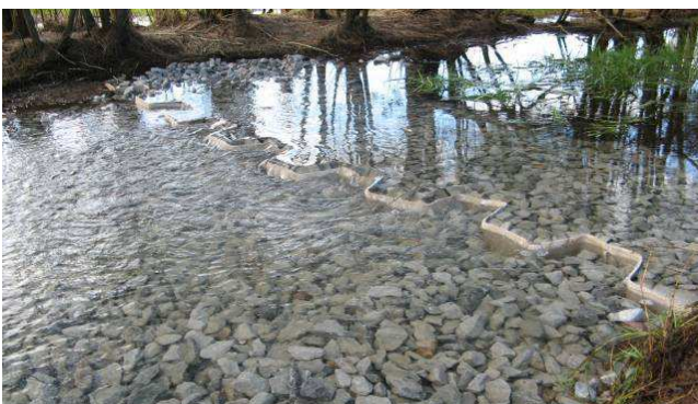
Image 39: vinyl sheet piling weir (S Murphy - Clarence Valley Council)
