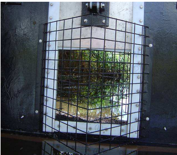
Image 67: square mesh debris shield (Photo: W Glamore, UNSW)
