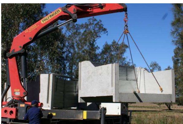
Image 56: installation of precast drop-board weir (S Walsh)
