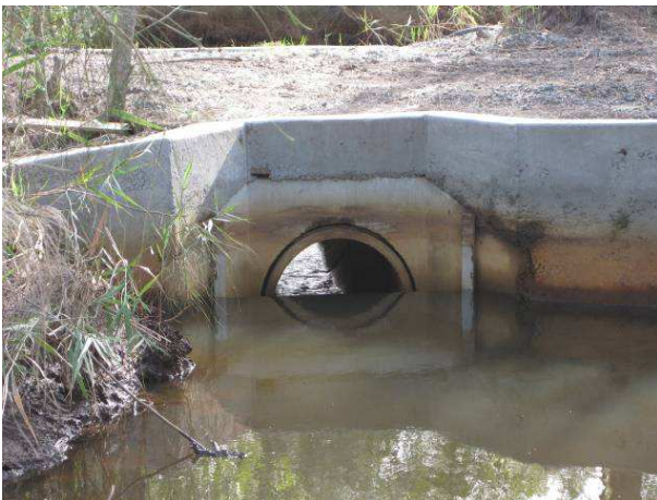
Image 51: drop-board culvert retrofitted to suit existing culverts in Anna Bay (K Russell)
