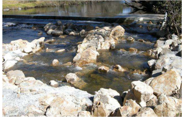
Image 70: rock ramp fishway installed about Higgin's Causeway in Gloucester
