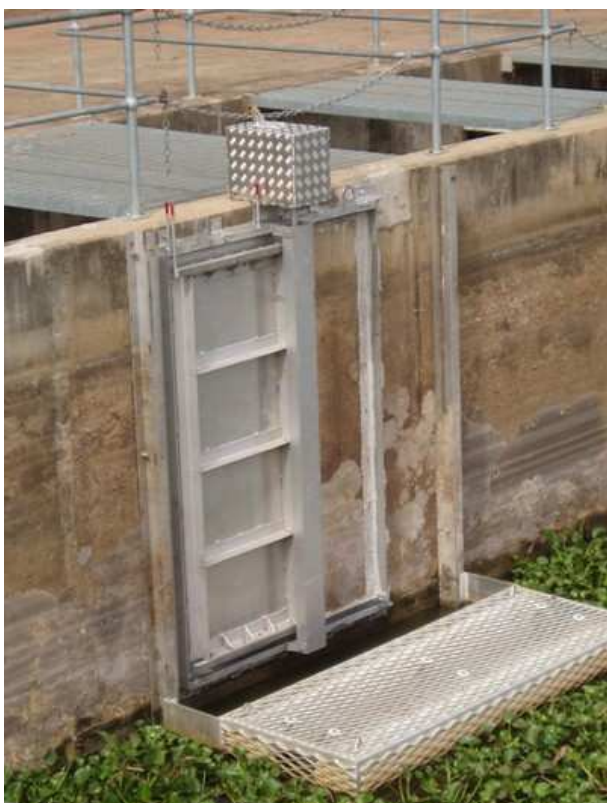
Image 62: sidewinder gate installed for SunWater QLD (AWMA)
