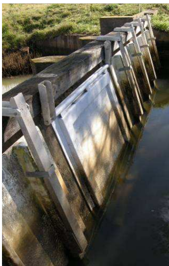
Image 33: fibreglass ballast gate in the Manning Valley
