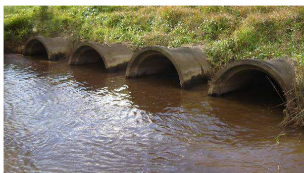
Image 2: multiple concrete pipe culverts
