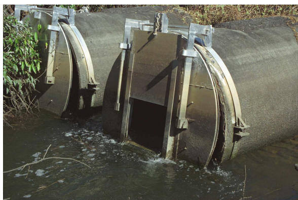
Image 25: sluice on a lockable chain system (S Walsh)
