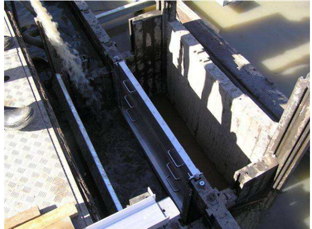
Image 40: solid plastic sheet piling weir incorporating drop boards for added functionality (Vonmac)
