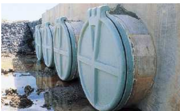
Image 11: fibreglass gates with neoprene seal (Humes)
