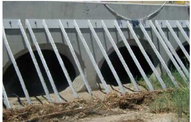
Image 68: steel debris rack (Photo: Bradley et al , 2005)
