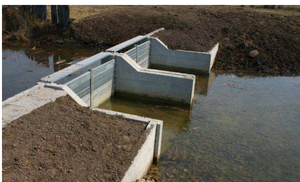
Image 58: installation of precast drop-board weir (S Walsh)
