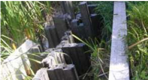
Image 37: v-section plastic sheet piling weir (Vonmac)
