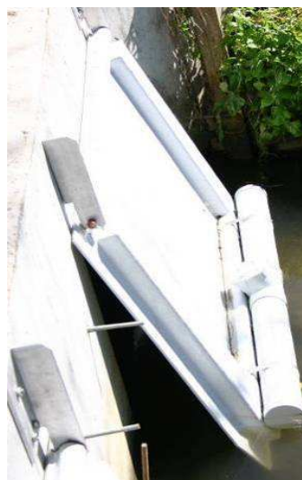
Image 34: fibreglass ballast gate in the Manning Valley (S Walsh)
