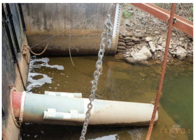
Plate 10 : Liquid levelling regulator
