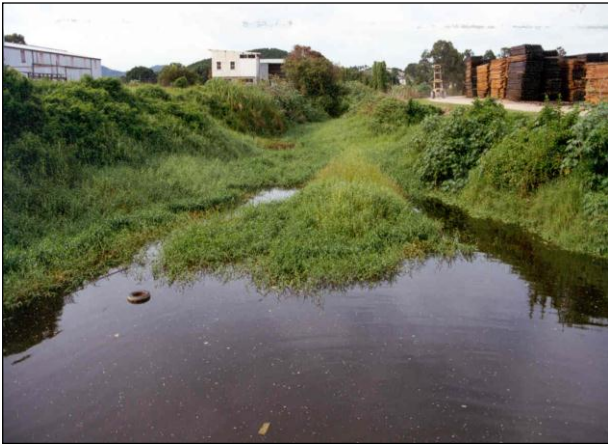
Plate 5: Before active floodgate management, Condong Creek (4/98).
