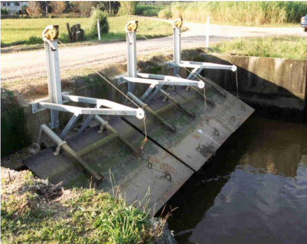
Plate 5: Installation of lifting devices (derricks and winches) on headwalls
