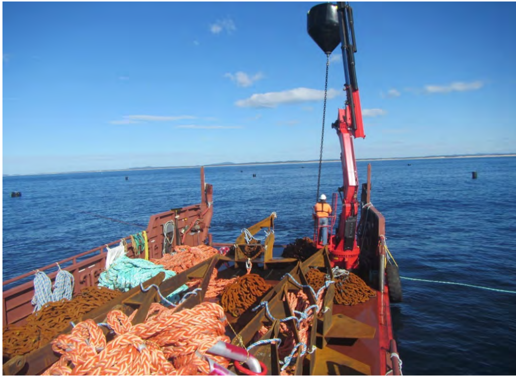
Figure 2: The deployment of anchors, anchor deployment lines and mooring lines on the MARL (Source: Huon, 2016).
