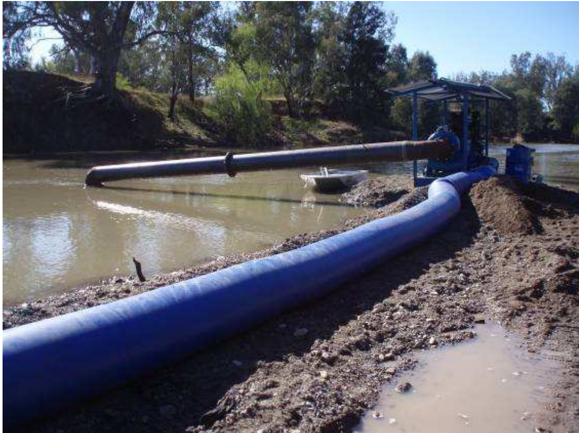
Figure 2. Picture of the experimental pumping station showing typical deployment into water adjacent to a gravel bar.
