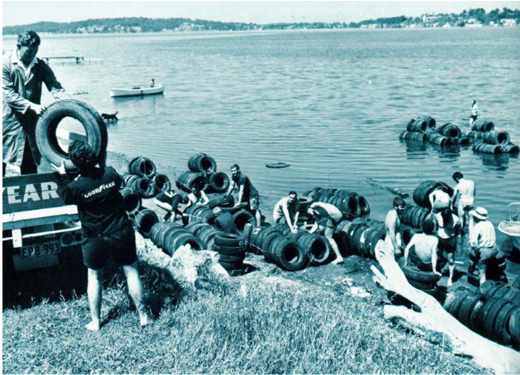
Figure 4. Initial deployment of artificial reefs in Lake Macquarie constructed from tyres.
