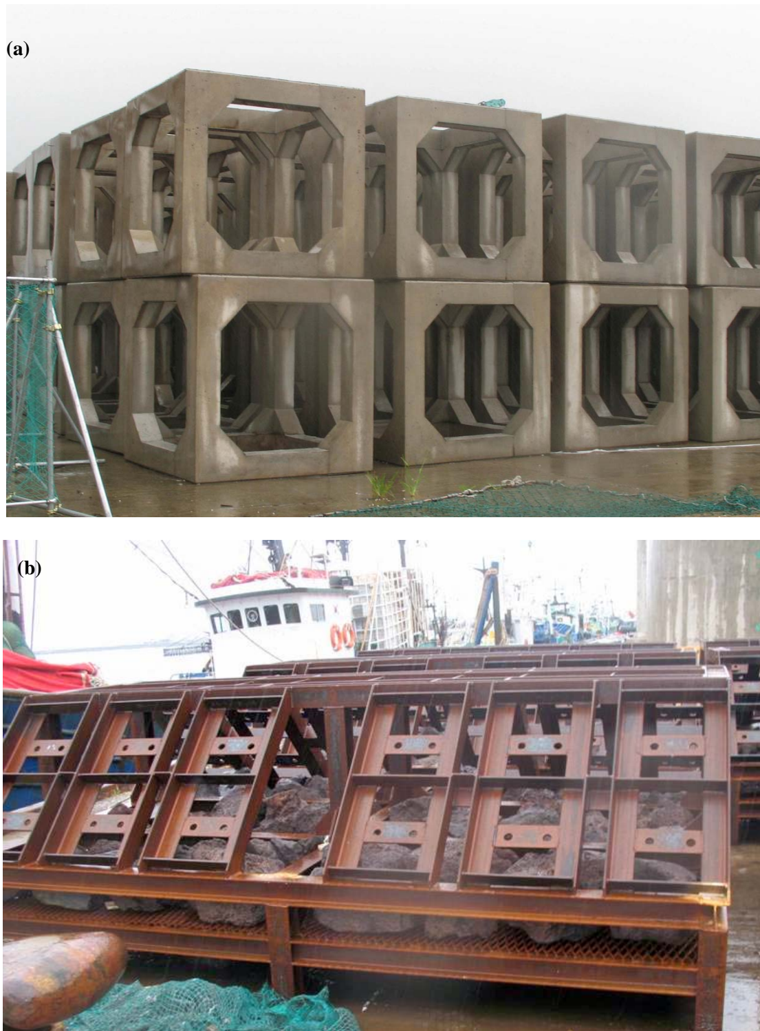
Figure 3. Examples of ‘design specific’ artificial reef units (a) individual concrete cubes for deployment in deeper water (20 – 40m) (b) steel reefs designed for abalone production at shallower depths (10 – 20m).
