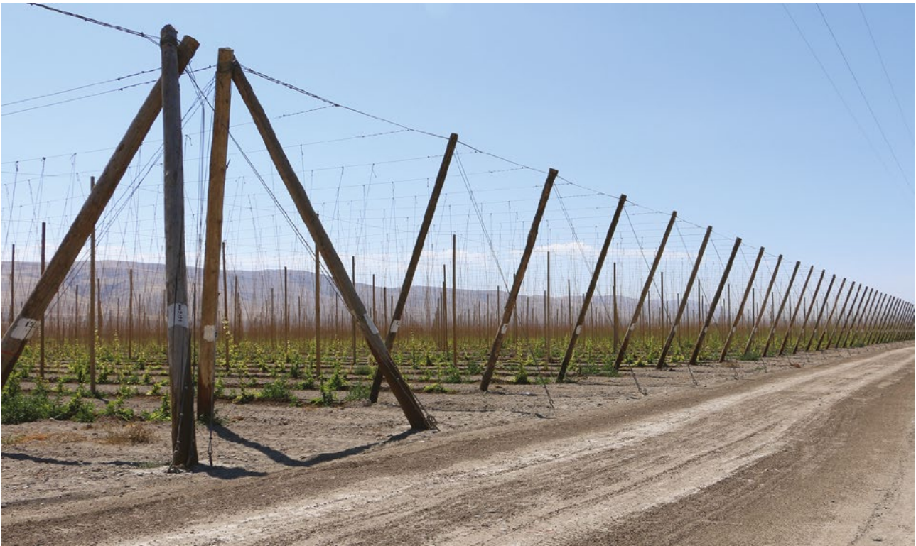
Figure 5. Image of a newly established 6 m V-trellised hop yard showing pole distribution, cabling, foliage wires and end assemblies (Yakima, USA).
