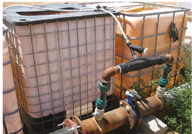
Figure 16. A basic fertigation injection system.
