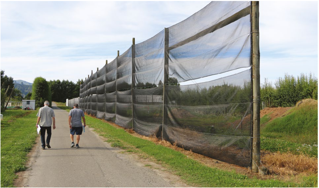
Figure 6. An example of a post and mesh shelterbelt on a site that is otherwise exposed to wind.
