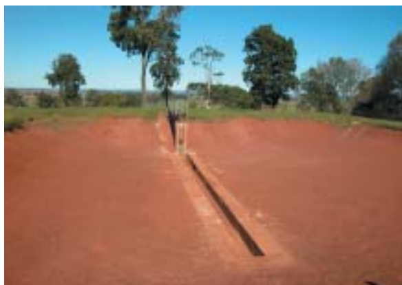
Fig. 6.4 Dry earthen pond showing the outlet tower and internal harvest sump.
