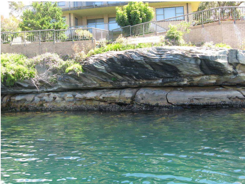
Figure 28. Vertical rock platform.
